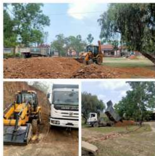
Earth filling and campus work
