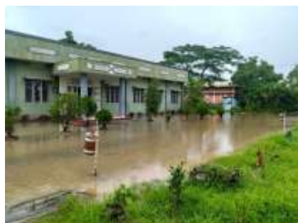
Flooded campus during July 2024
