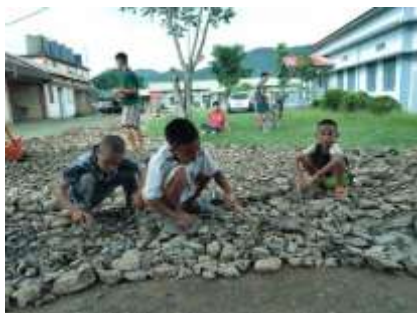
Approach road work
